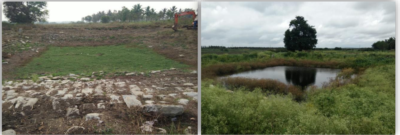
Kalyani in Shantigramma, Hassan taluk & District, before and during Rejuvenation
