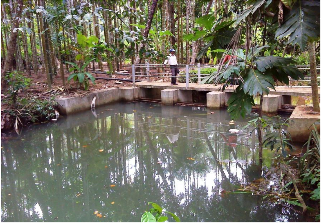
Vented Dam in Mavalli, Bhatkal Taluk, U.K District
